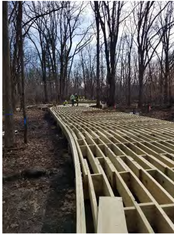
Setting deep supports and making the curves: overlapping and bending support joists
