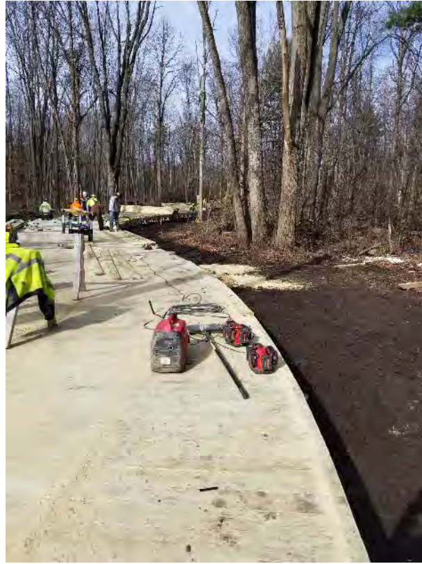
Making the curves: ripping deck boards on an angle and trimming sides after screwing on deck boards
