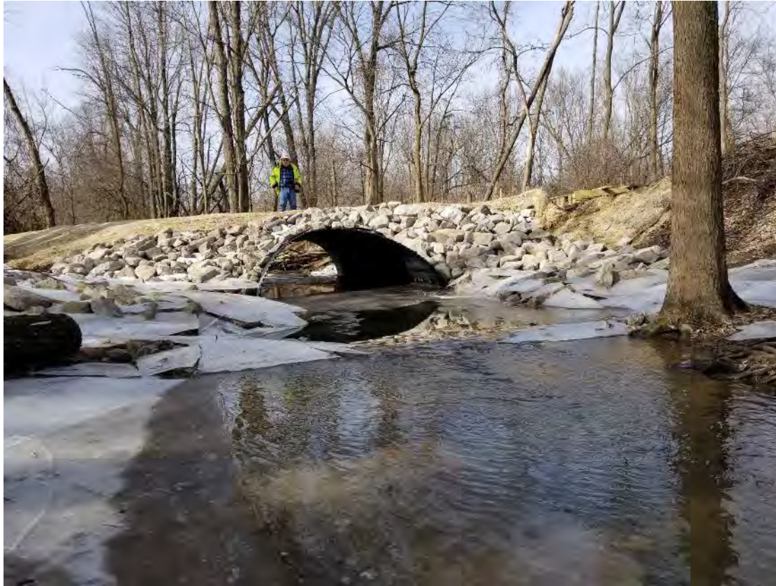
Culvert on Lucas Drain with downstream grade control riffle. (Mark Goss from Spicer for scale!)
