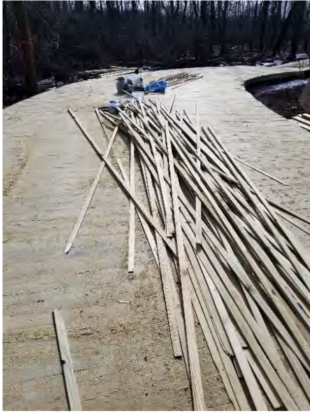
Making the curves: ripping deck boards on an angle and trimming sides after screwing on deck boards
