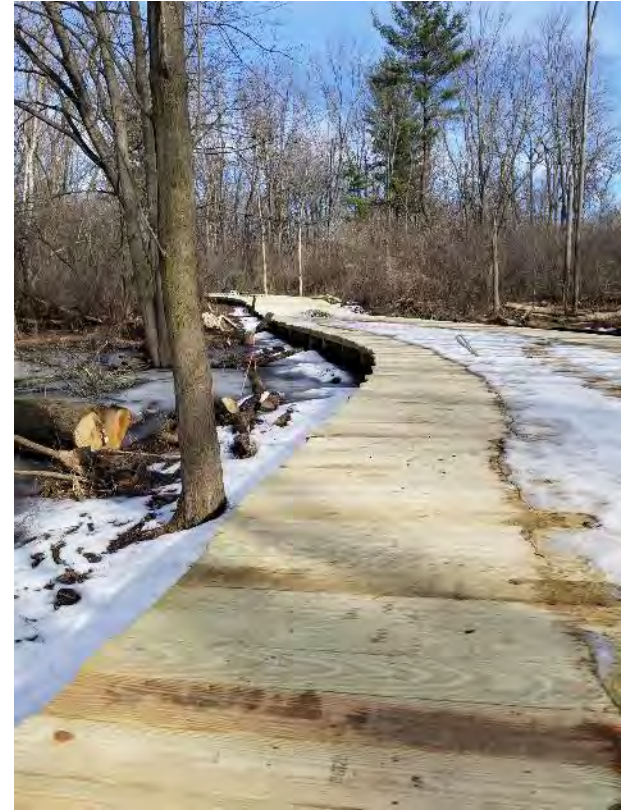
Making the curves: ripping deck boards on an angle and trimming sides after screwing on deck boards
