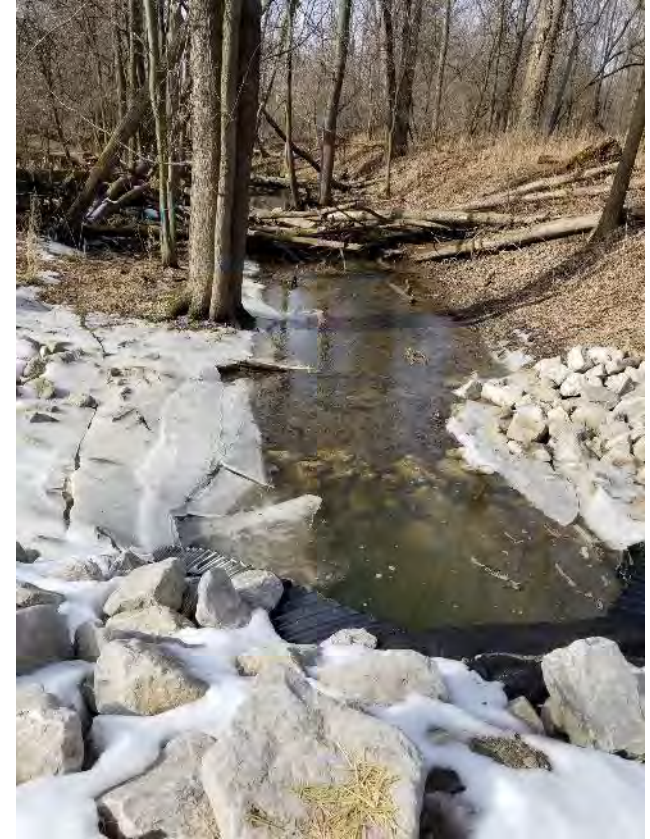
Culvert on Lucas Drain with downstream grade control riffle. (Mark Goss from Spicer for scale!)
